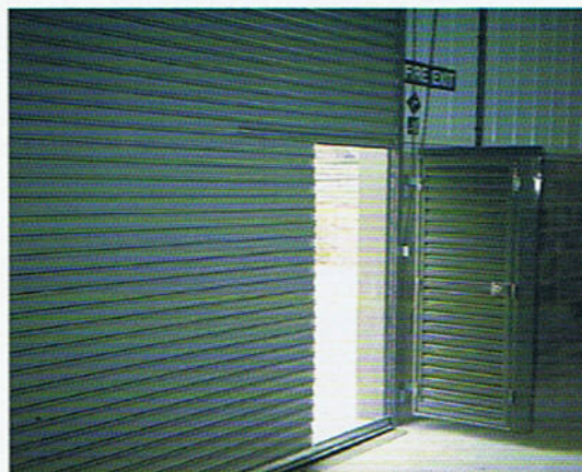
Wicket Door with frame hinged clear to allow operation of Rolling Shutter.
