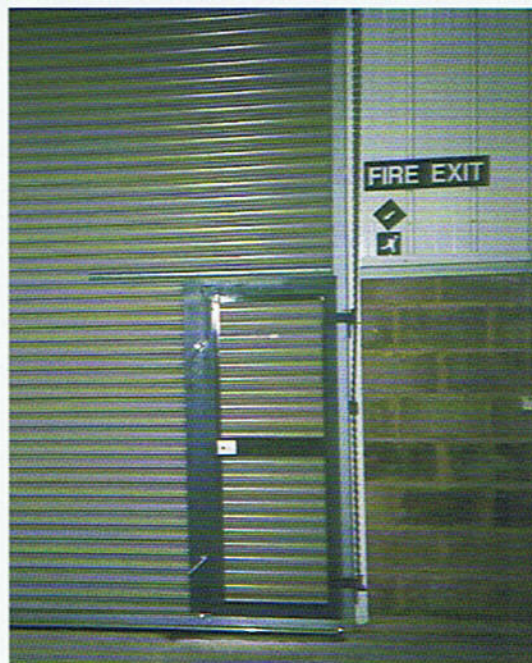
Wicket Door in secured position.
