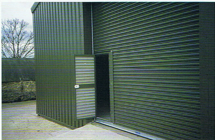
Wicket Door open for access.
